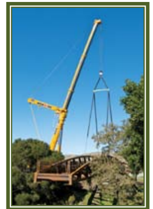
New Bridge Fernandez Ranch
